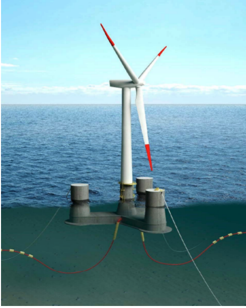
(a) OO-Star Wind Floater applies a concrete foundation [15]
