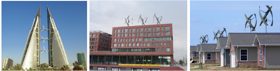
Figure 1.6: From left to right: Bahrain World Trade Center with building integrated wind turbines ( Atkins, 2008 ), Roof-mounted wind turbines on the Greenpeace headquarters in Hamburg ( Neuhauser, 2016 ), stand-alone turbines besides houses in residential area in Illinois ( EcoPlanetEnergy, 2011 ).
