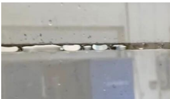
Figure 4.4: A partial water bridge in the lower joint. Photo taken during test no. 58 with Fiber Cement White panels and a 5 mm joint width.
