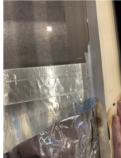
Figure C4: To avoid water intrusion behind or on the outside of the gutter system the top of the gutter is taped with aluminium tape and the sides are sealed with a waterproof sealant.
