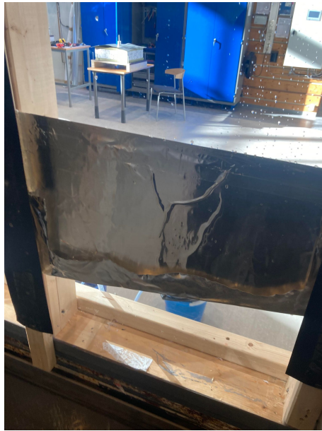
Figure C5: After a test measurement the gutters were improved by cutting them so that the edges did not touch the panels, and thereby get more water than they should.
