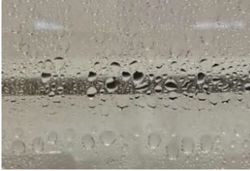
Figure 4.6: Direct spray through the top joint to the wind barrier. Photo taken during test no. 86 with Fiber Cement White and an 8 mm joint.
