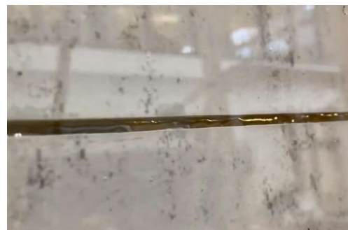
Figure 4.5: Water bridge that is continuous throughout the lower joint. Photo taken during test no. 43 with Fiber Cement Grey panels and a 3 mm joint width.
