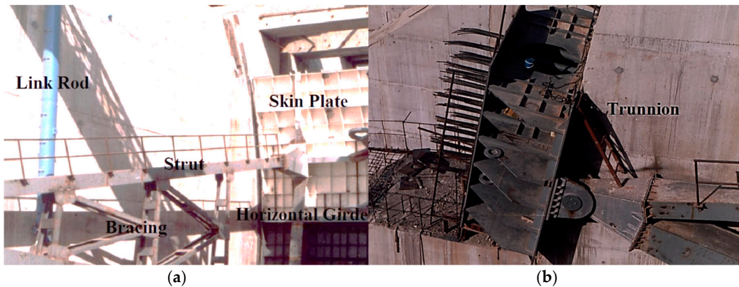
Figure 2. Primary radial gate components of Karkheh Dam (a) truss and skin plate, (b) trunnion beam.
