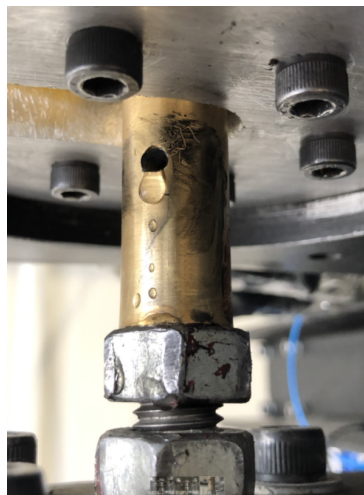
Figure 15.9: Water flowing through safety outlet.
