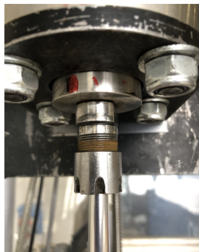
(b) Drill pipe connection leading to leakage.
