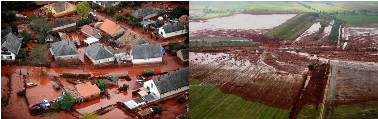
Figure 2. Pictures of the flooding of Devescer (left) and the breach of the holding pond in Ajka (right) 17 , ©MTI.
