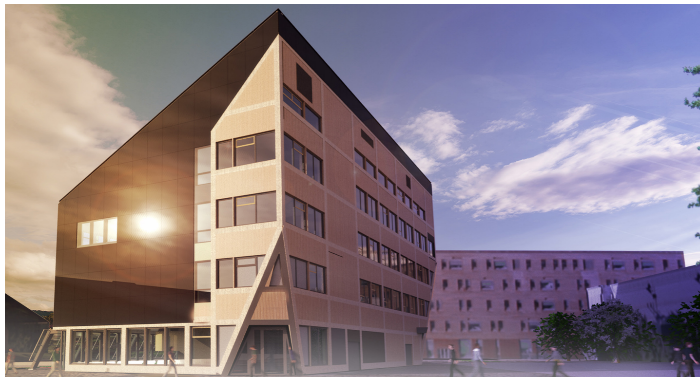
Figure 1: ZEB Laboratory building. Illustration: LINK Arkitektur
