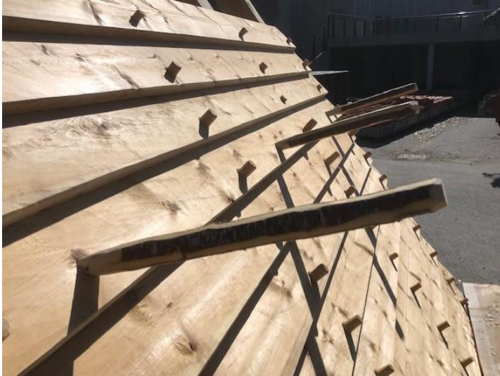
Figur 92 Naglar i bjerk for stillasplank
