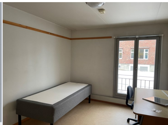
Existing window 1.2mx2.0m
