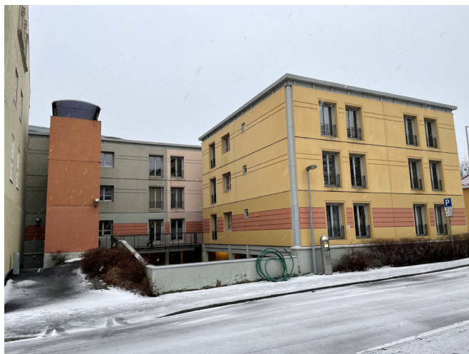
West Facade along Schwachs gate
