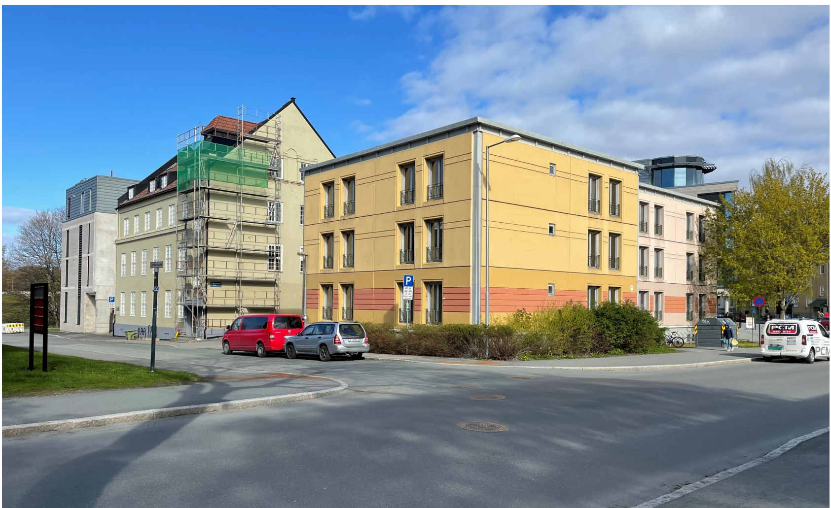
Existing facade along Klostergate
