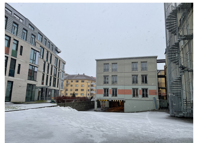
North Facade facing Nidelva
