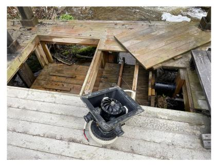
Figure 65: Hydro Turbine Generator Placement
