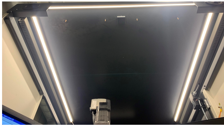
Figure 25: New lighting on the ceiling.
