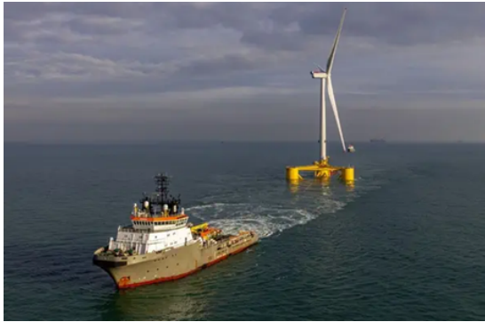
Figure 5.11: A tug vessel dragging a floating wind turbine in constructing the Kincardine wind farm [77]
