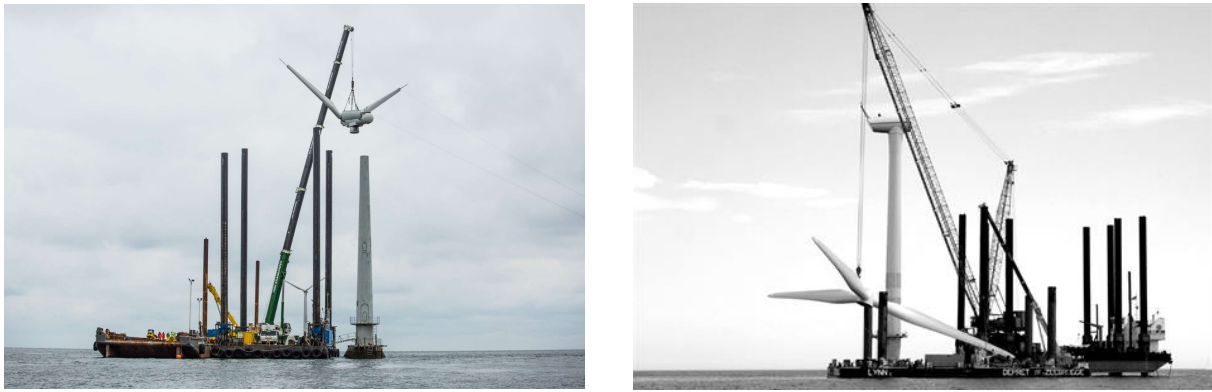
Figure 5.14: Decommissioning of an offshore wind turbine [95, 96]
