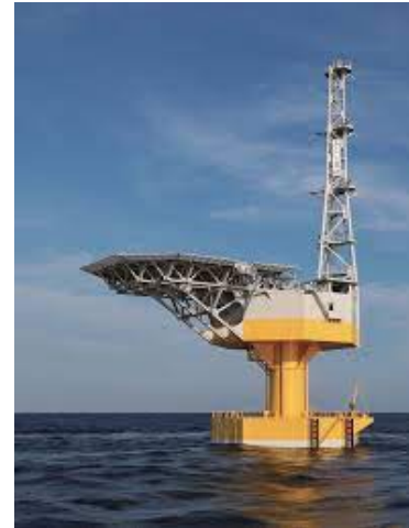
Figure 5.10: Floating offshore substation, Fukushima Kizuna [74]
