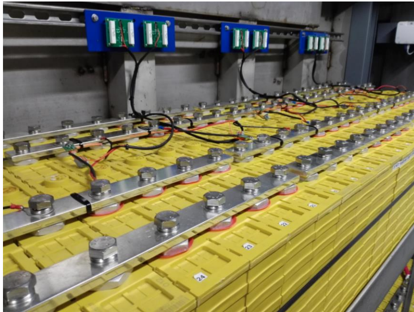
Figure 2.13: LFP cells connected in parallel and series. Source: Wikimedia Commons [18]
