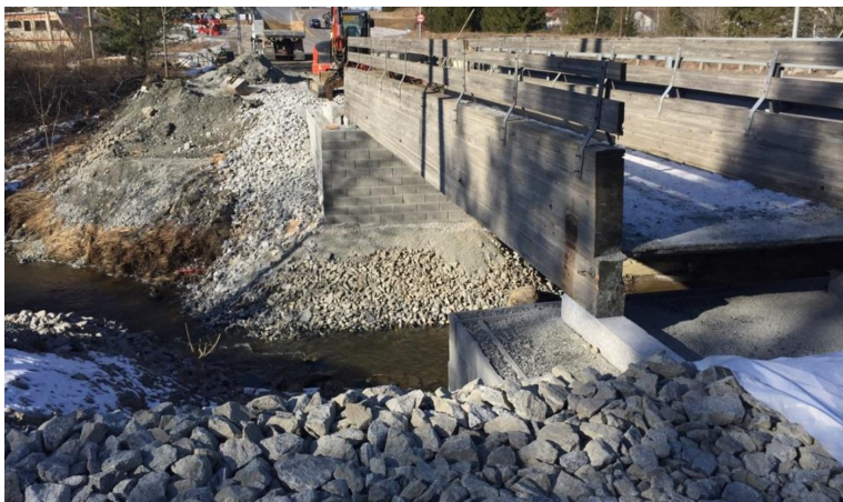
Figure 1.3: Kråkstad pedestrian bridge, constructed using GRS abutments (Vaslestad and Anthi, 2017).
