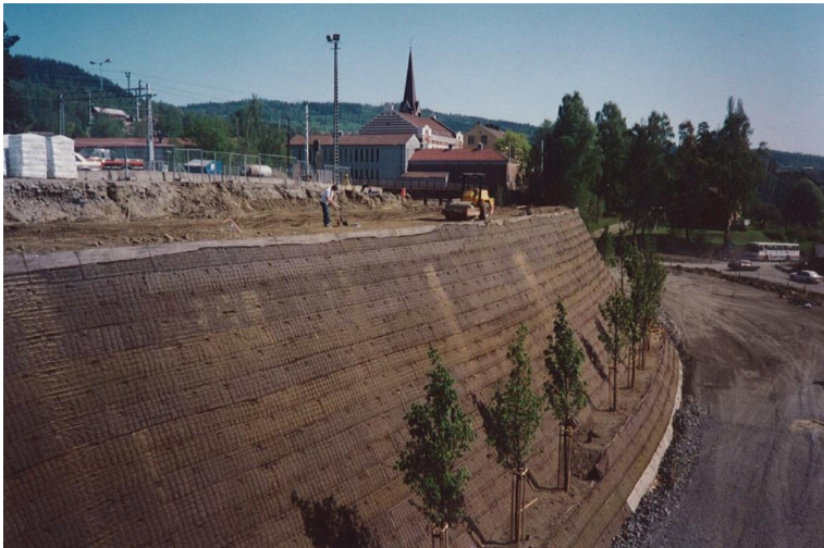
Figure 3.9: Picture of the finished slope, not yet vegetated (Vaslestad et al., 1996)
