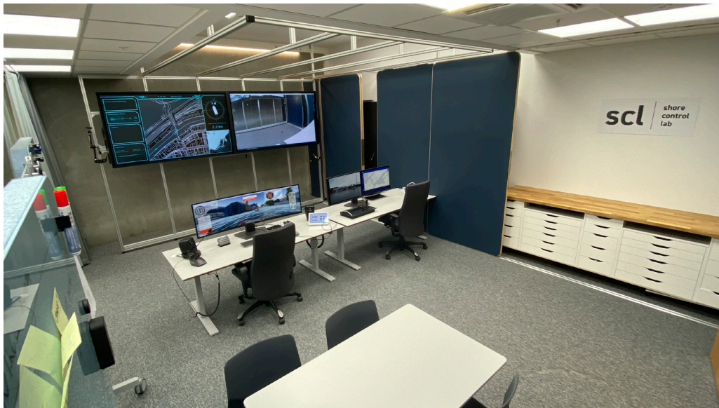
Image: The control room located at the SCL headquarters. This is where operators monitor autonomous vessels from.
