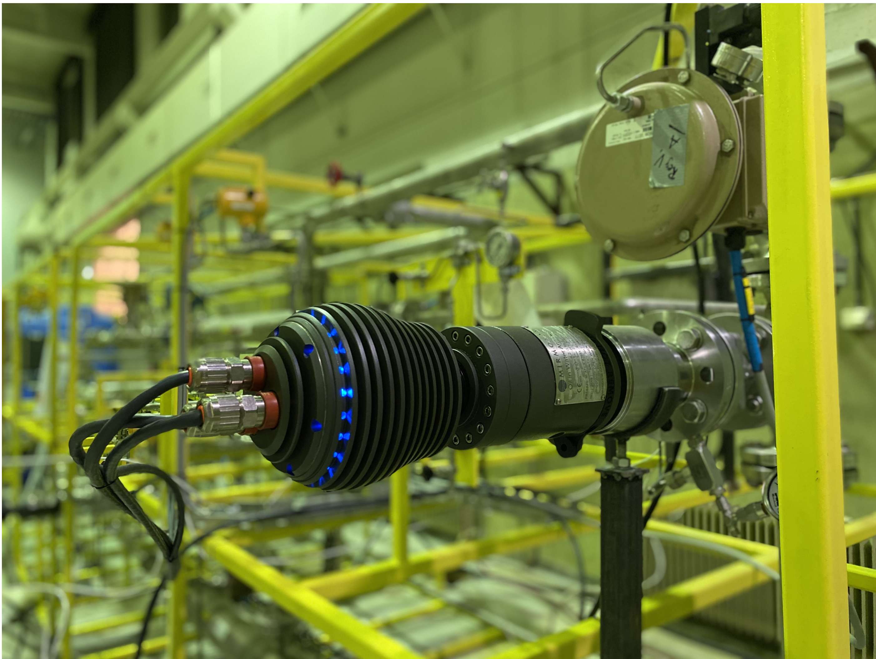
Figure A.2: Mirmorax online oil-in-water analyser installed at the test-rig.
