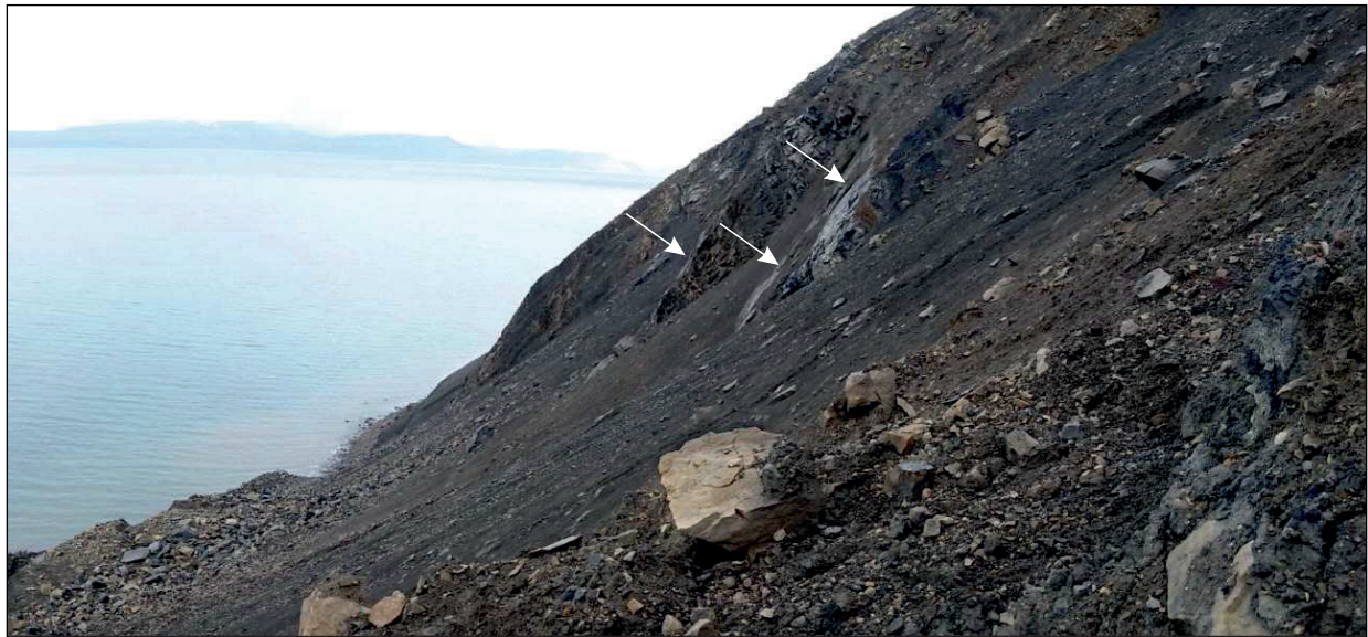
Figure 14. Active gravitational mass wasting along the coastal scarp of Block 13. Instability along adversely oriented slide surfaces (orientation: 26/55 NW) are a consequence of basal sea-cliff erosion and slope oversteepening. White arrows indicate slope-parallel sliding surfaces, view towards north.
