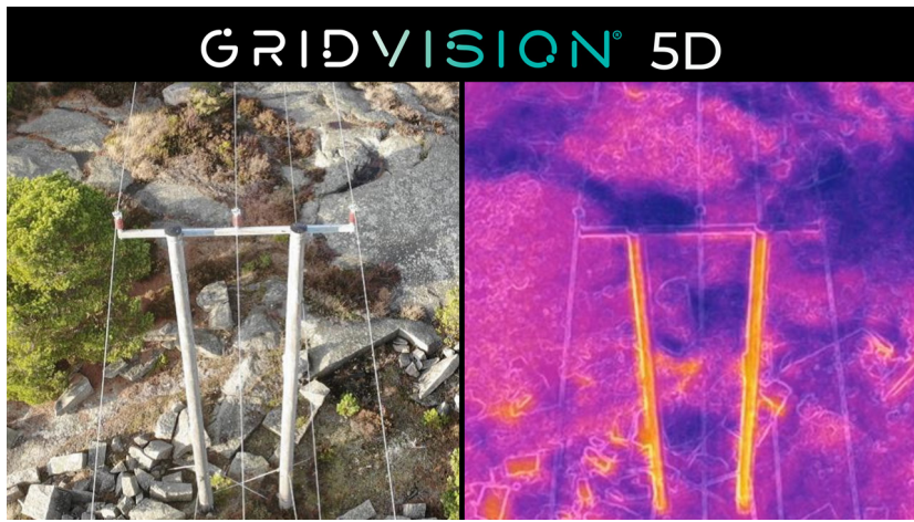
Figure 1.3: GridVision5D Photo: eSmart Systems
