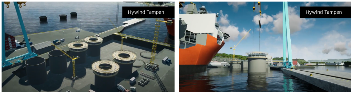
(a) Slipforming in dry dock
