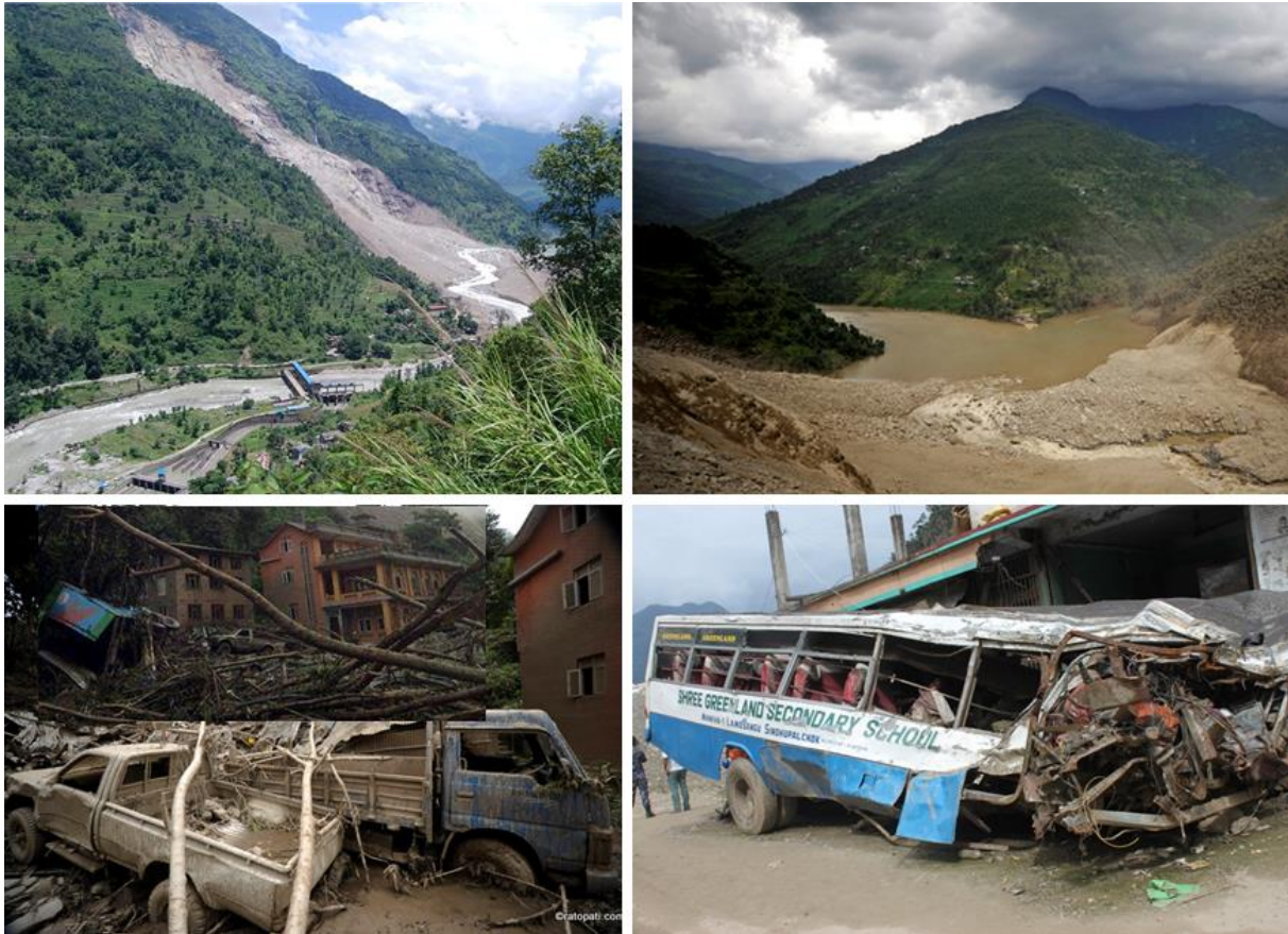
Figure 4. Jure landslide, damming of Sunkoshi River and damages caused by landslide.
