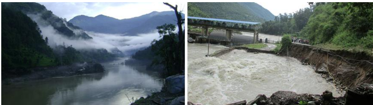
Figure 5. Lake formed by the landslide (left) and damage to road and headwroks of Sunkoshi HPP.
