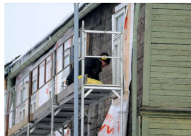
Figure 8. Renovation of the façade (Trondheim Municipality, 2016).
