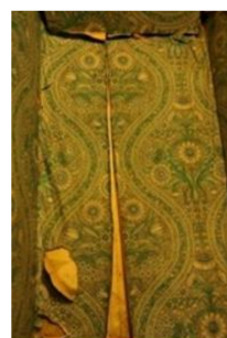
Figure 12. Indoor wall in one of the rooms (NTNU).
