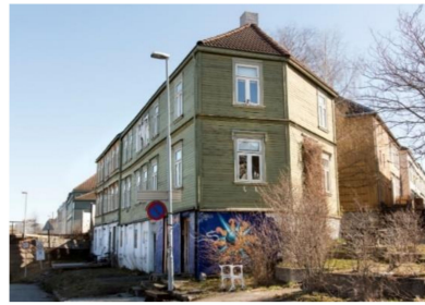
Figure 7. Strandveien 19 and 21 (Trondheim Municipality, 2016).
