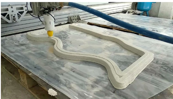
FIGURE 3. Pipe delivering printing material (3D Cons project).
