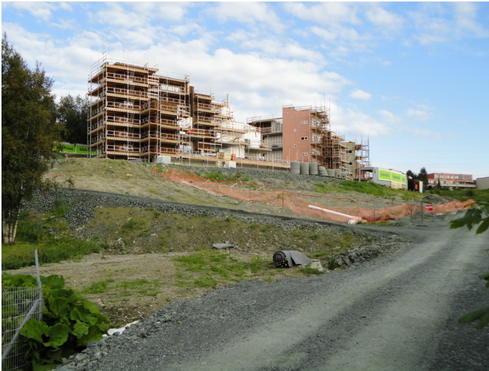
Figure 66: Construction of 27 new apartments, date taken: 23.08.2011
