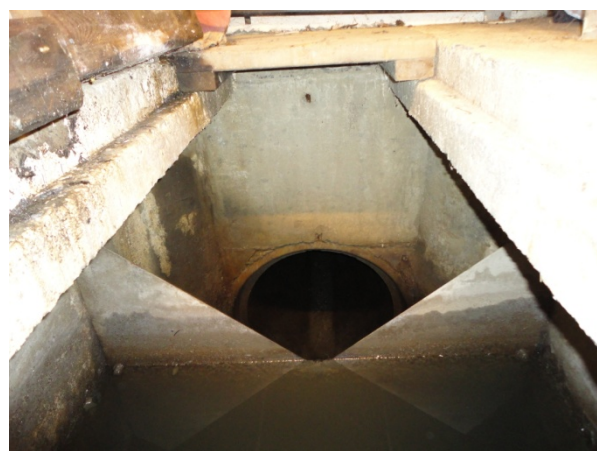
Figure 77: The V – notch weir from another angle
