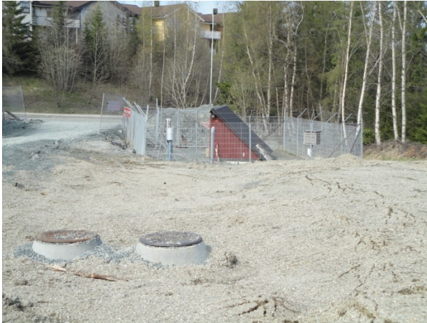
Figure 46: Location of replaced manholes
