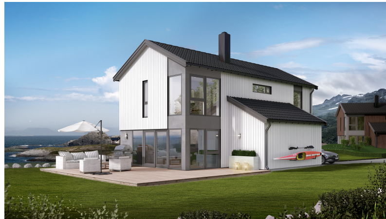
Figure 5. Case building representing a typical residential building in Norway (source: Norgeshus).
