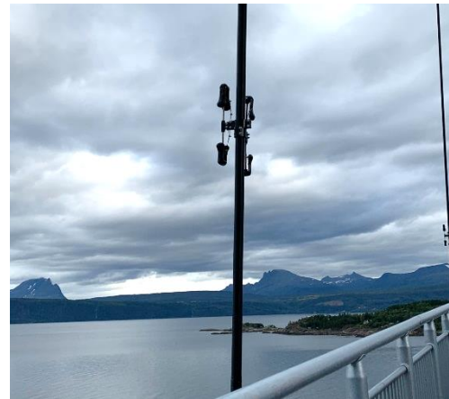
Figure 5. Stockbridge damper mounted on hanger.
