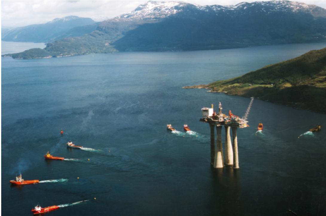
Figure 2: Troll A towage in 1995 (Norcem, 2021)
