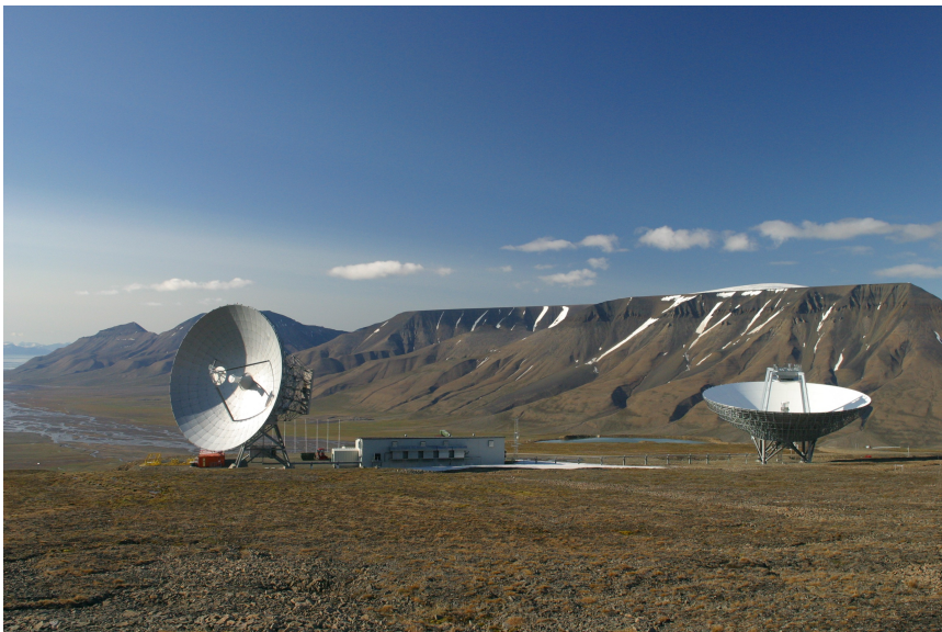
Figure 3.7: Picture of the EISCAT Svalbard Radar, with the 32m dish pointing towards the south on the left and the field-aligned 42m dish on the right. Figure courtesy of EISCAT.
