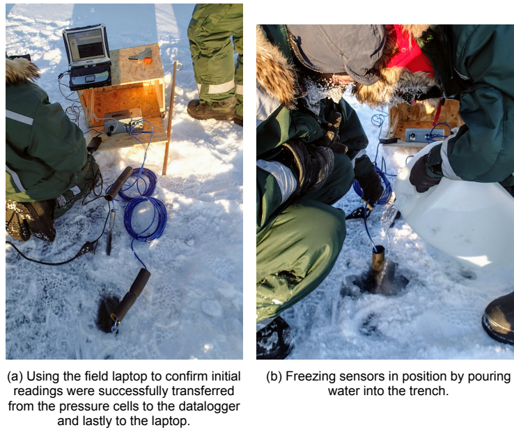
Figure 3.20: Svea fieldwork equipment installation.
