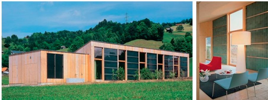
Fig. 1. On the left; External view of building with a combination of standard windows and PCM-windows (Architekten, 2000a). On the right; internal view of standard windows and PCM-windows in combination, PCM being the semi-translucent elements on the sides of the windows (Architekten, 2000b, 2004).
