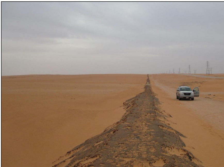
Figure 9-1: Field-D TL-12 Onshore Pipeline
