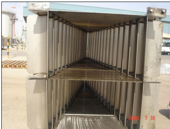
Figure 6-41: Multi-Vane Inlet Type at Field-B GOSP
