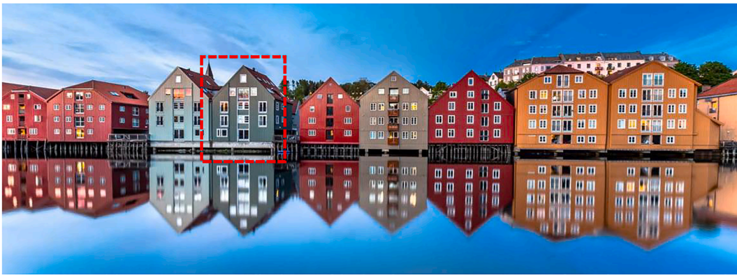
Fig. 29. Selected renovation building by Nidelva river (inside the red dash frame). (For interpretation of the references to color in this figure legend, the reader is referred to the web version of this article.)
