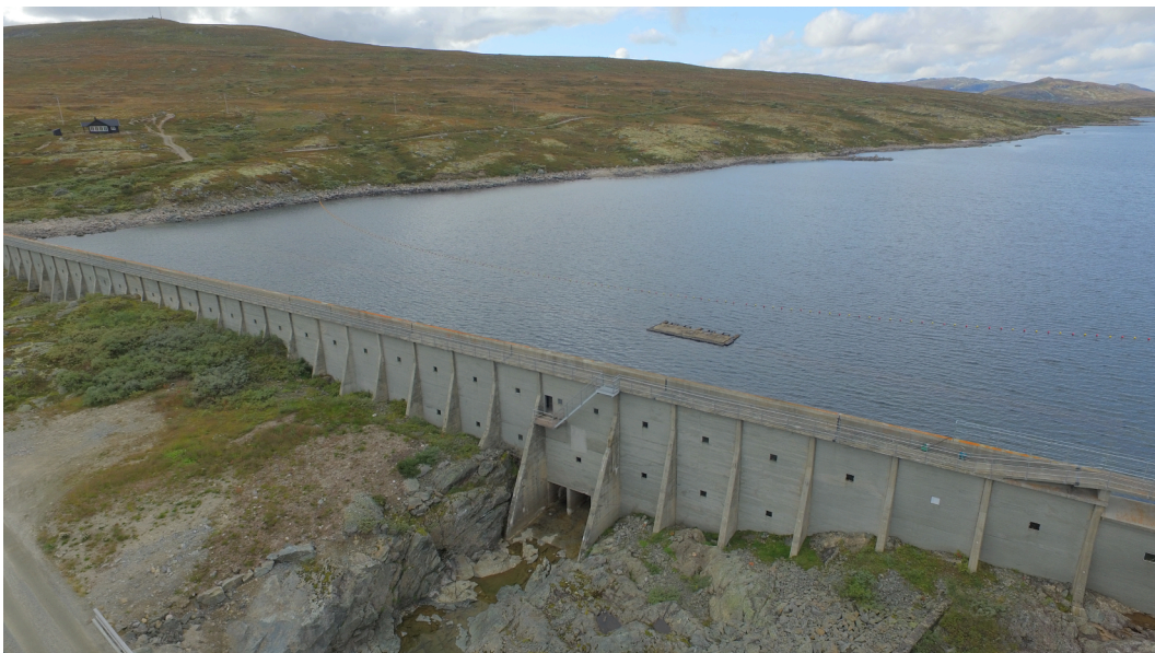
Fig. 1. Overview of Kalhovd dam.
