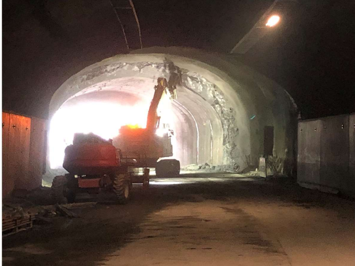
Figure 7-1. Pigging of concrete vault in tunnel rehabilitation.
