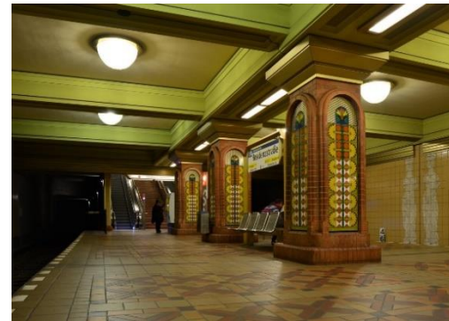
Figure 4 Massive pillars blocking clear view of the station at U Residenzstraße (Fiedler, 2018)
