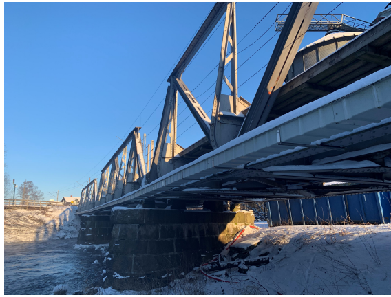
Figure 4.3: Picture of Sokna Bridge.
