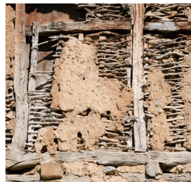
Figure 2-13: Wattle and daub wall. Source: (MrPanyGoff, 2012)
