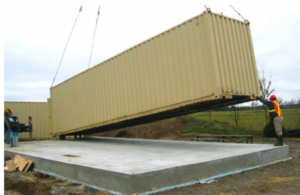
Figure 2-10: Shipping container on mat foundation. Source: (Sanchez, 2021)
