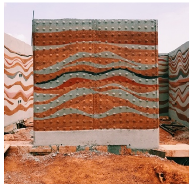
Figure 2-12: Rammed earth construction. Source: (Hive Earth, 2018)
