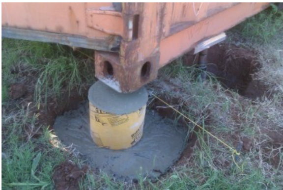
Figure 2-9: Shipping container on spread footing foundation Source: (Premier Box, 2017)
