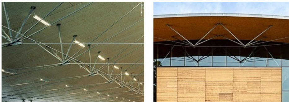
Figure 5.1: V-shaped spacious compression rods of (1) Flyinge Ridhus, and (2) TU Graz timber lab
