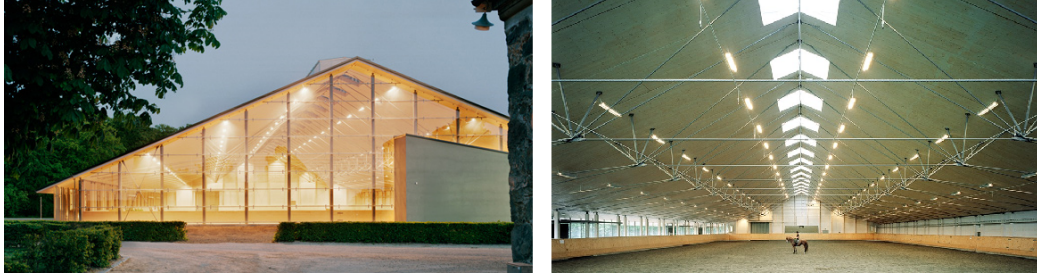
Figure 1.2: The under-spanned CLT roof of Flyinge Ridhus
