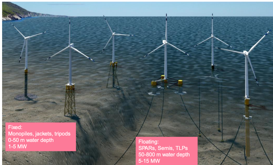
Figure 2.2: Foundations used in offshore wind industry (Equinor, 2020)
