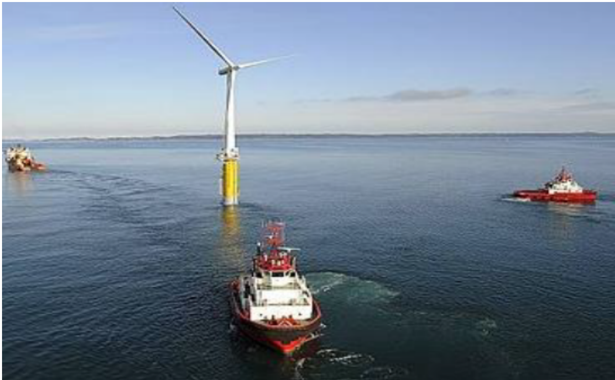
Figure 3.4: Towing operation in Hywind Scotland project (Lien, 2016).
