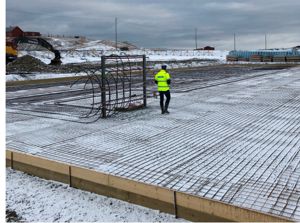
(b) 17.09.2020; placement of cooling pipes.
