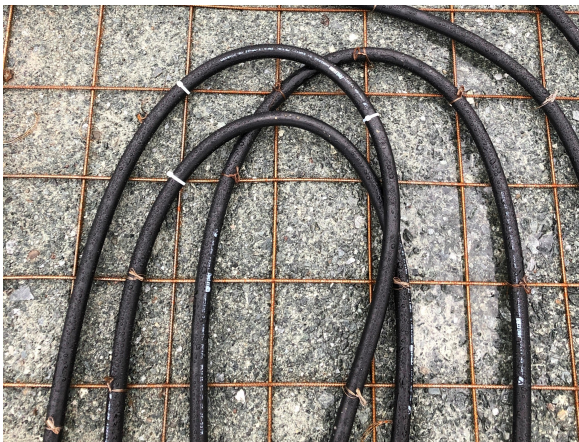
(c) 28.09.2020; fixing cooling pipes to reinforcement.
