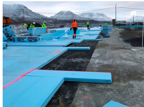
(f) 12.10.2020; placement of XPS insulation.
