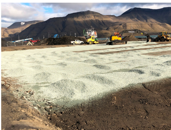
(c) 19.08.2020; clean base layer on top of compacted fill.
