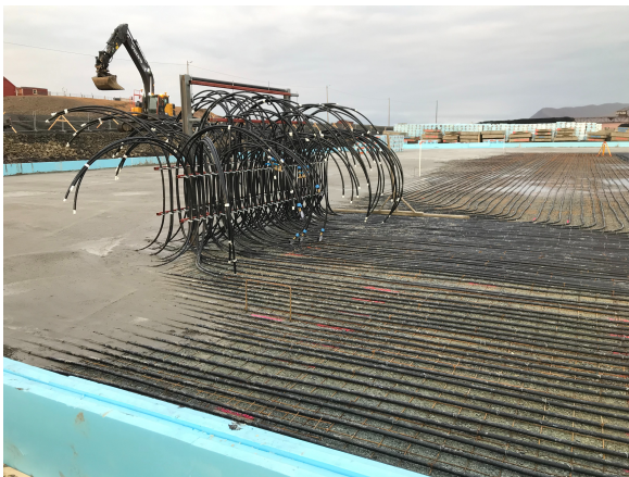
(e) 05.10.2019; outlet for cooling pipes and casting of concrete.
