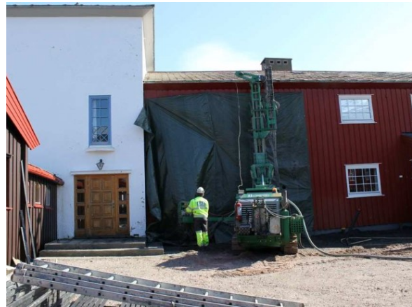
(b) Reconstruction of the Sysselemandsgården foundation (Rongved and Instanes, 2012).
