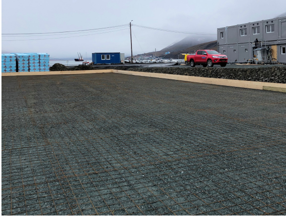
(a) 14.09.2020; placement of reinforcement bars.
