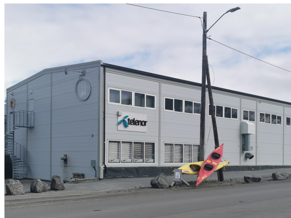
(f) Former ISS building (Photo taken by the author).
