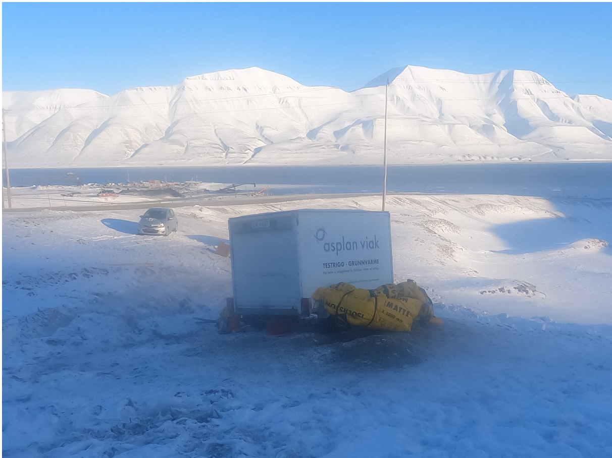
Figure 4.9: TRT rig at drill site 1.
