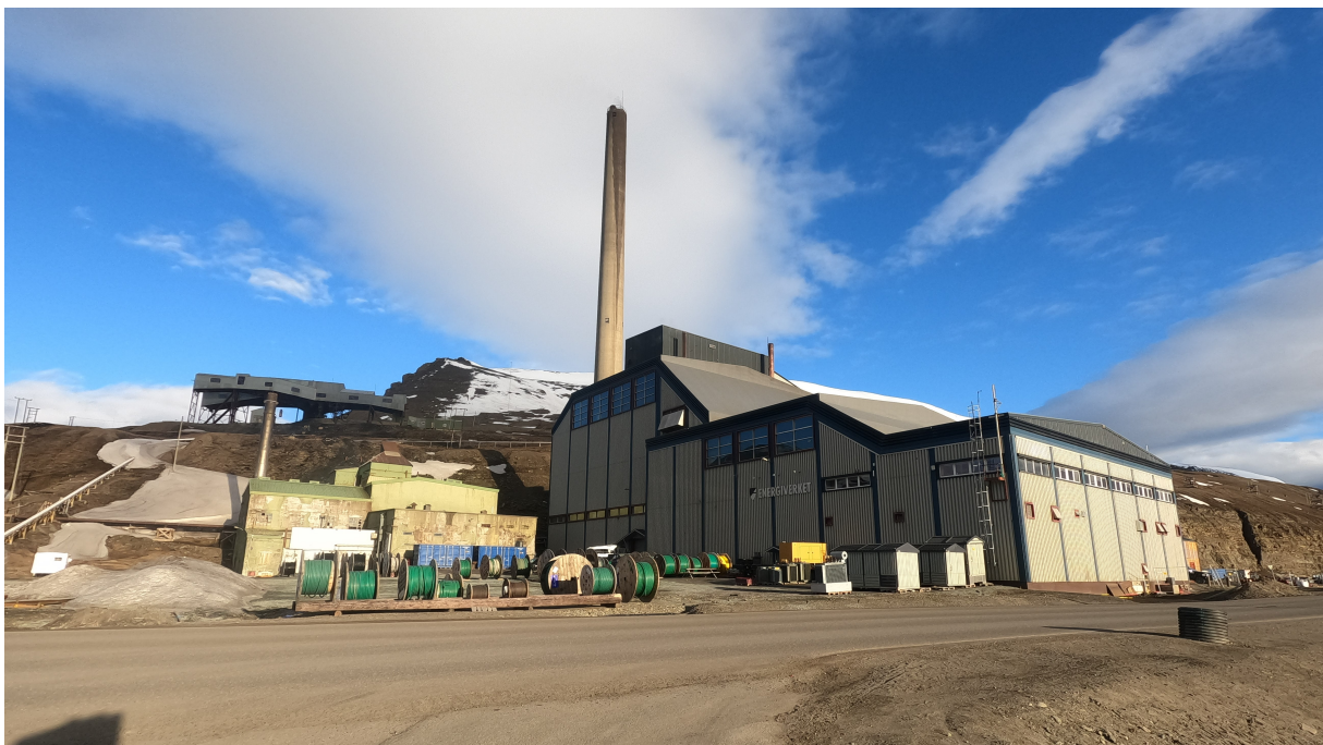
Figure 2.1: Coal powered CHP power plant in Longyearbyen. The old power plant can be seen on the left side of the picture.
