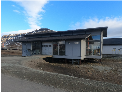
(a) Boiler station.
