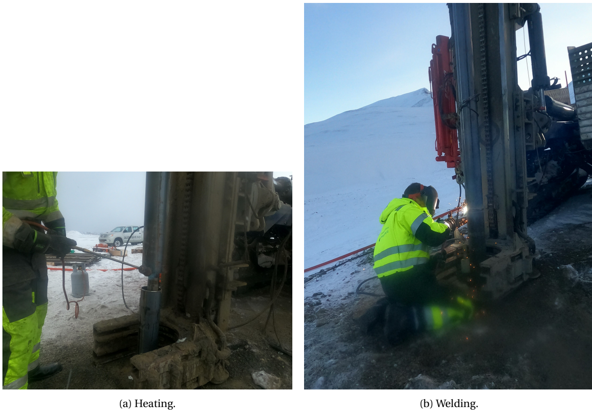
Figure 4.2: Heating and welding for extending of a soil casing.
