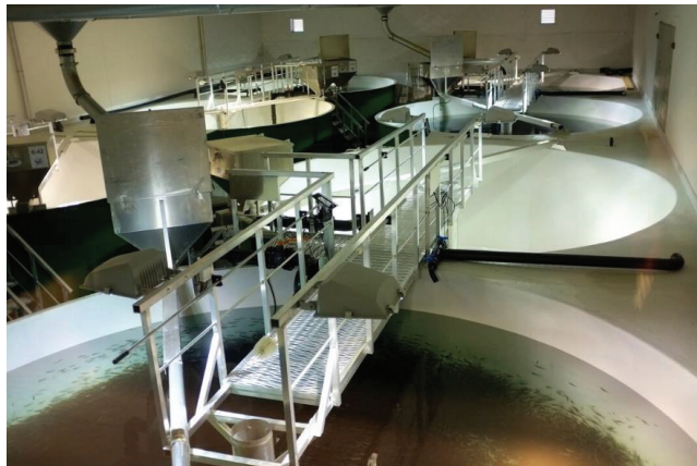
Figure 4. Juvenile salmon production in a RAS system (Photograph: Smolten AS, courtesy of the Norwegian Seafood Federation).
