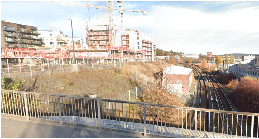
Figure 3.3: Photo from the side of the metro line and construction site. The picture is a screenshot from "Google Earth".
