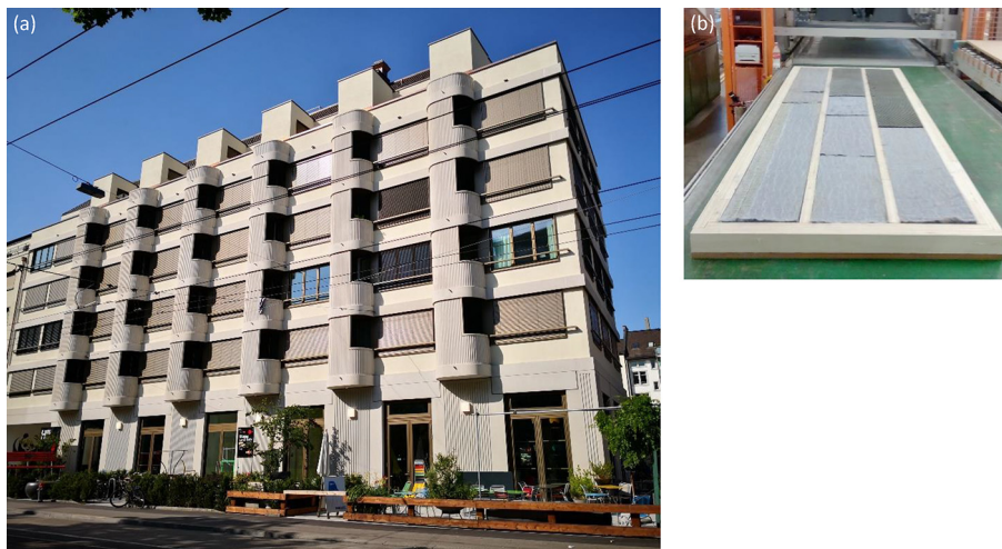
Fig. 12. First new building in Switzerland with aerogel insulation on the whole façade, located in the centre of Zurich. (a) View from the street with aerogel insulation under and next to the windows. (b) Assembly of aerogel façade element with grey aerogel blankets. Images: Jannis Wernery.
