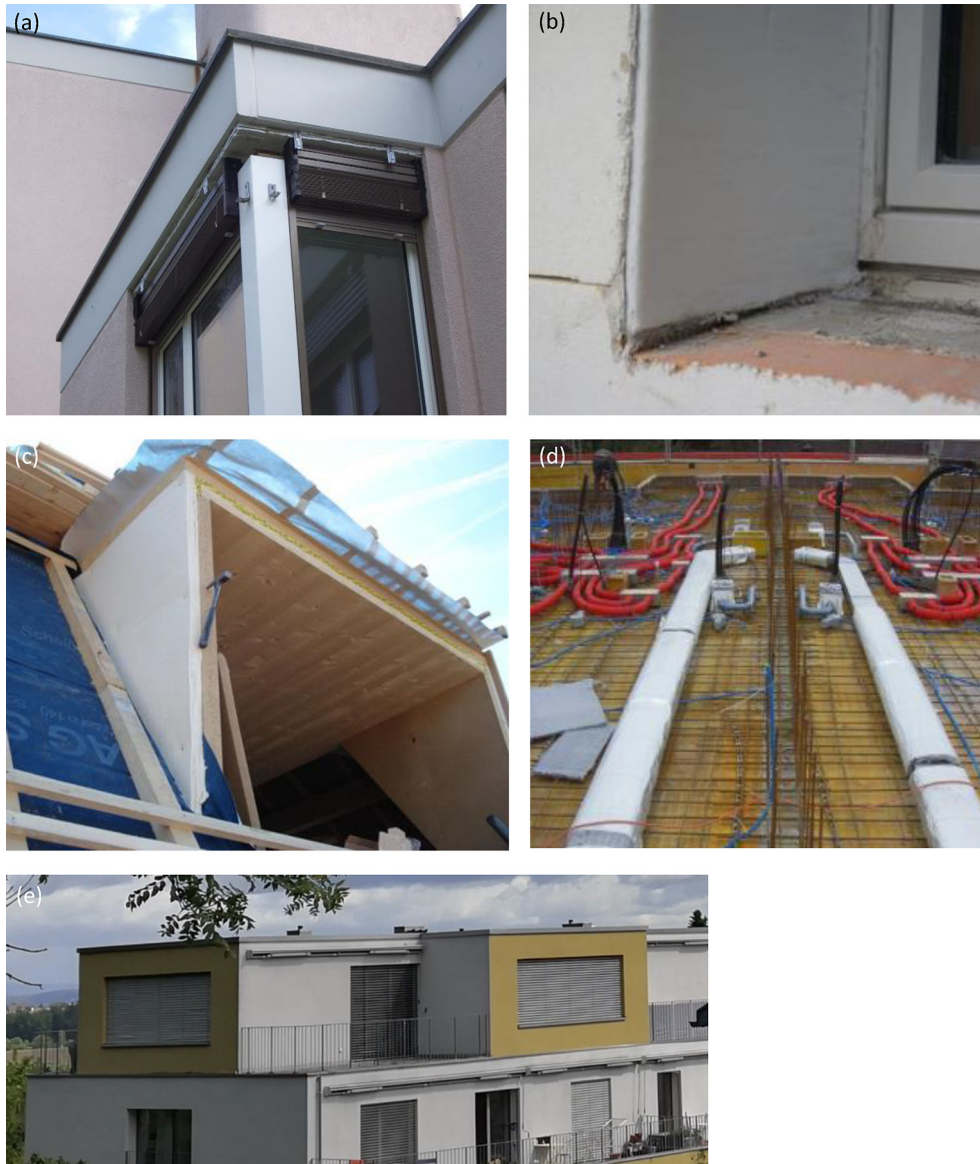
Fig. 3. Examples of architectural details where the use of superinsulation provides additional benefit compared to conventional insulation: (a) Roller shutter housing insulated on top and behind with silica aerogel blankets. (b) Silica aerogel insulation on window reveal: the thin layer avoids covering the window, whereas the façade is outfitted with conventional insulation. (c) Dormer window wall is insulated with silica aerogel (next to the hammer) in order to maximise window size. (d) Ventilation ducts in a ceiling before concrete pouring, insulated with silica aerogel (white). (e) Penthouse terrace. Images: (a)-(d): AGITEC AG, (e) Jannis Wernery.
