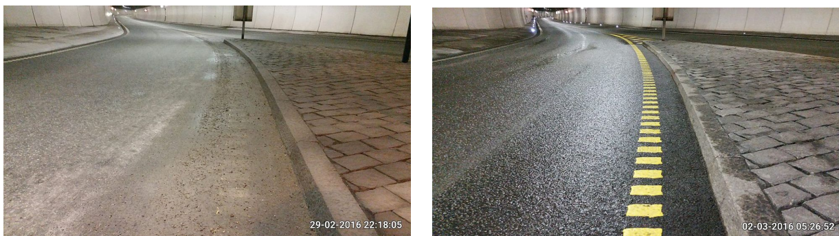
Figure 1: Illustrative tunnel road surface before and after wash, showing improved visibility of road markings. Photos: Norwegian Public Roads Administration, Trondheim 2016 (Midtbø, 2016).
