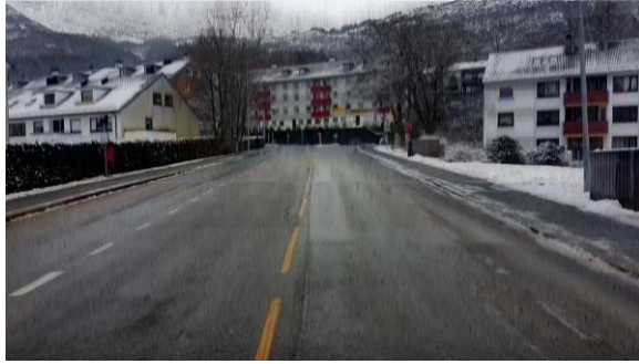
a) Intersection 1 and the western approach
