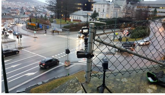
a) Mounting of the northernmost cameras at intersection 2
