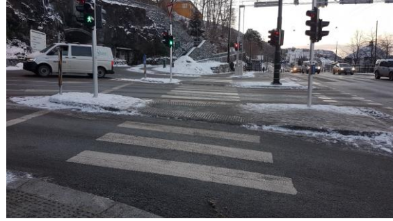
b) The pedestrian crossing is divided into three parts on the eastern approach
