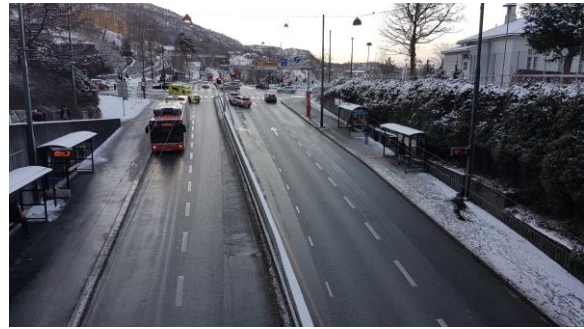
b) The intersection seen from the northern approach
