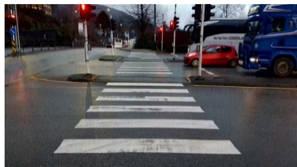
d) The pedestrian crossing is divided into three parts on the western approach
