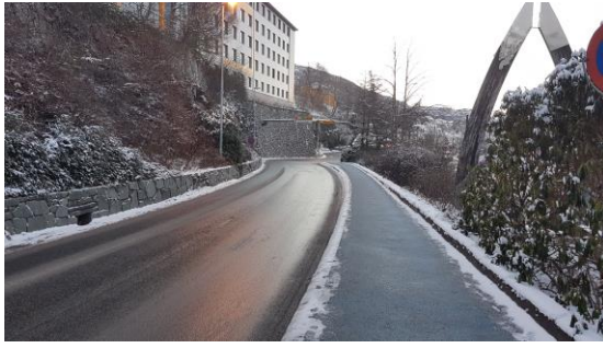
a) The road leading from Haukeland University Hospital to the intersection
