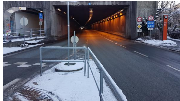
d) The other side of the tunnel on the northern approach
