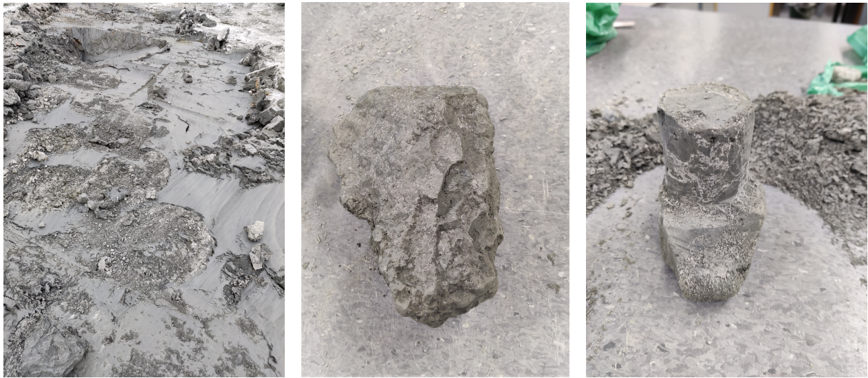
(a) Contours of lime-cement columns, visible between non-stabilised clay (b) Typical raw sample piece of stabilised clay (c) Trimming process of a field sample (F25 II)
