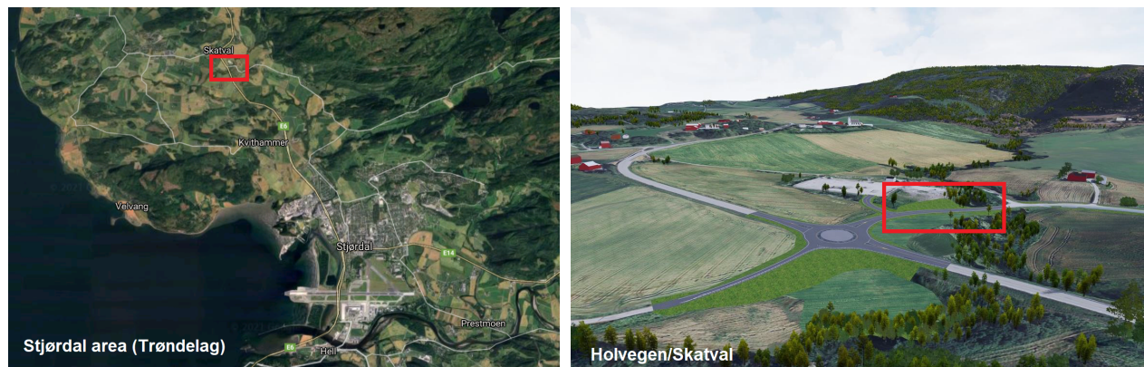
Figure 3.4: Map and model of the area for field stabilisation. Retrieved from Google Maps and Nye Veger (2020)
