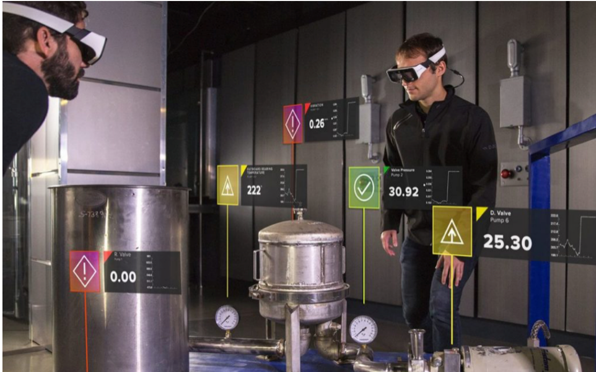
Figure 1 augmented reality for maintenance (Google)
