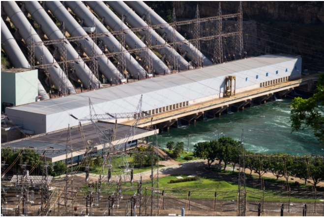
Fig. 2. A Picture of a Furnas hydropower plant in Brazil [8].
