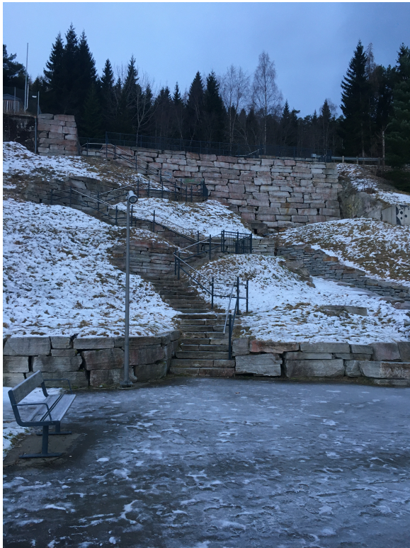
(a) Parts of the new Killingdal Park.
