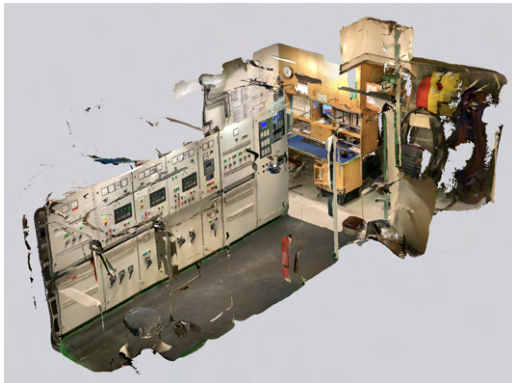
(e) LiDAR scan of the model explored in the Outside Engine Room, i.e. control room scene.
